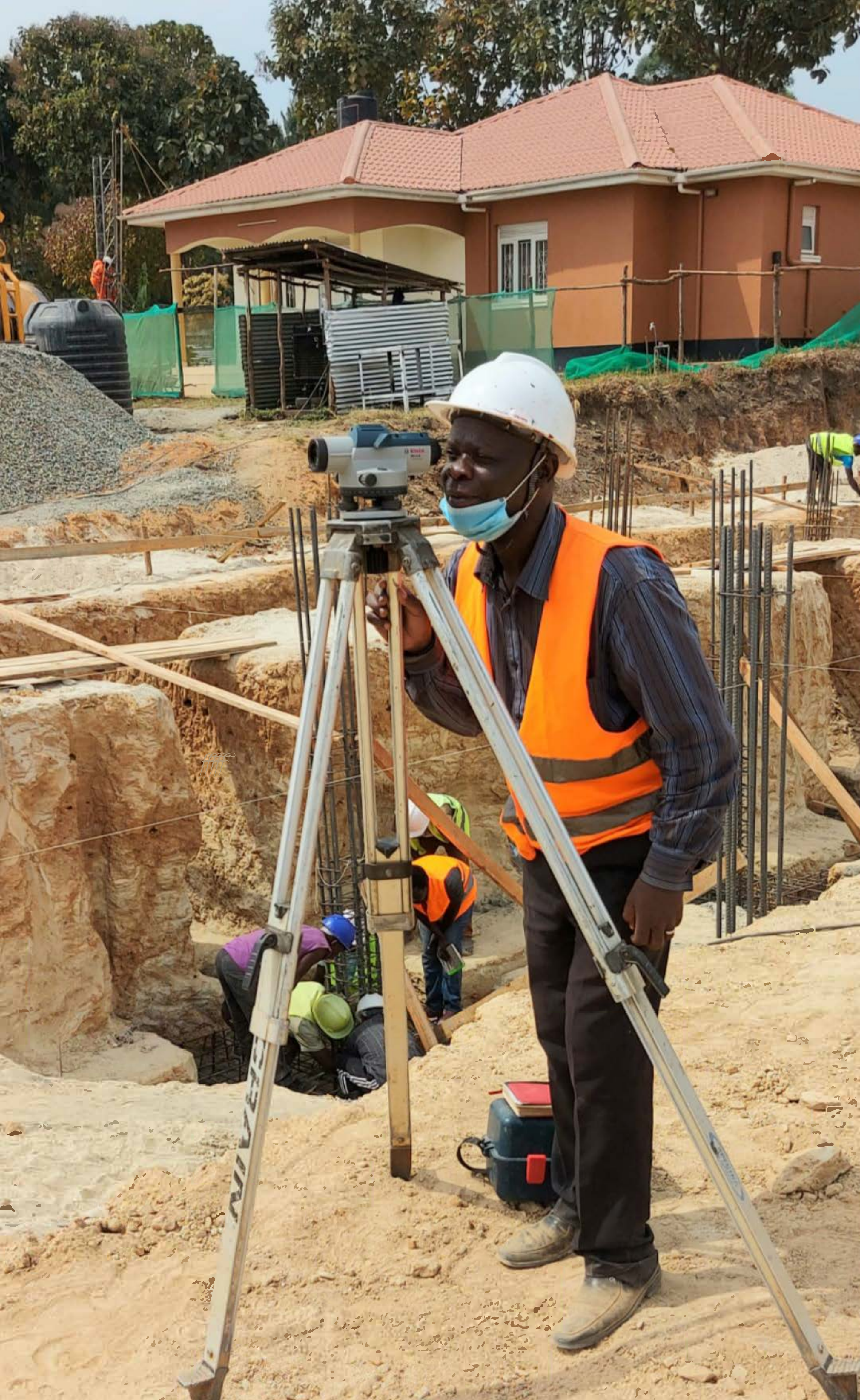
Wansa engineers at work on one of their sites
